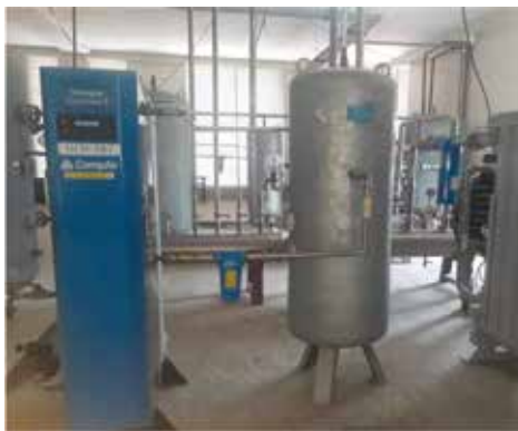
Nitrogen generator piping works
