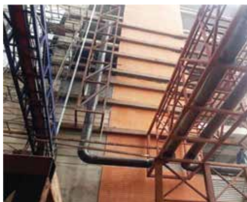
MS Pipe Bridge
