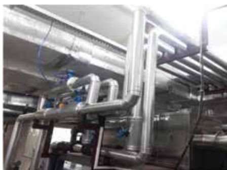
Chilled Water Piping works
