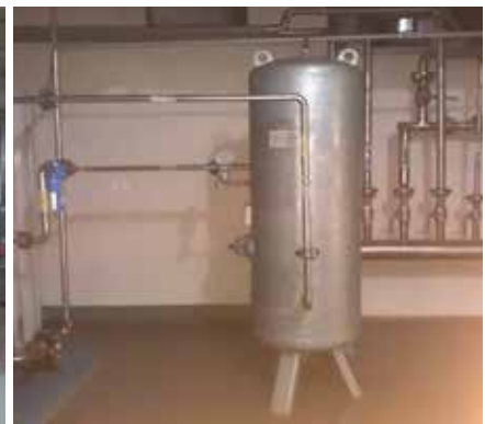
SS Piping Works
