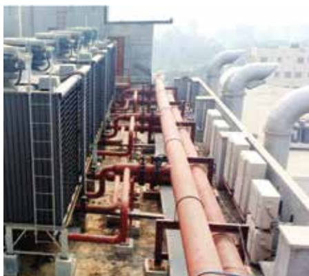
MS Piping Works
