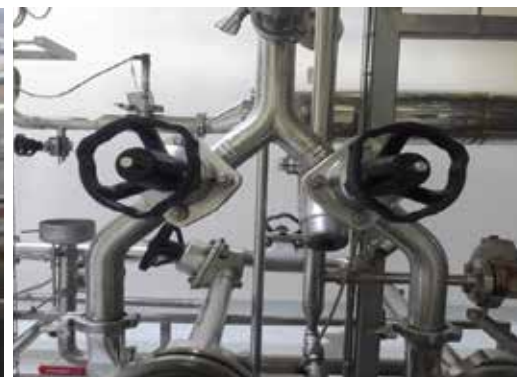
Process Line Piping Welding (SS 316L)
